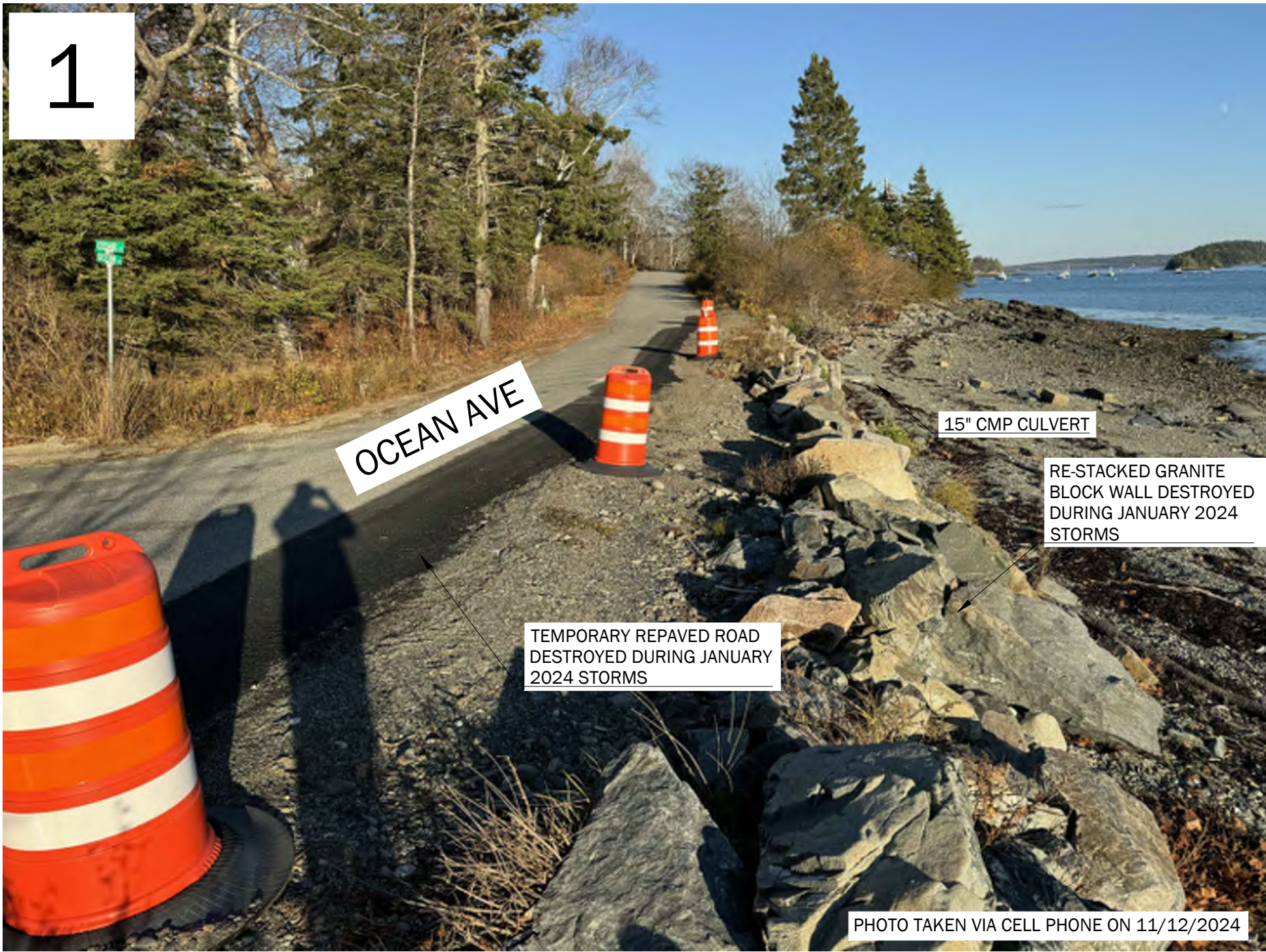
TEMPORARILY REPAIRED ROADWAY EROSION
